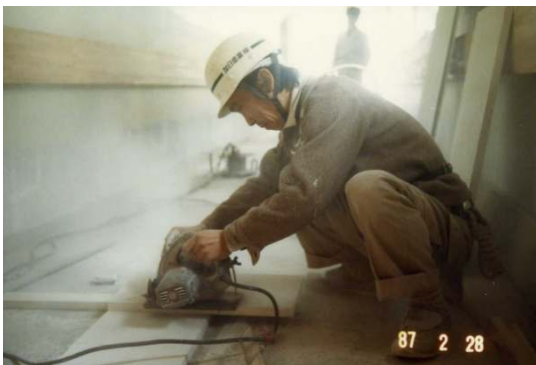
Fig.5. A carpenter cutting a board containing asbestos by an electric circular saw without mask. The airborne asbestos concentration in his respiratory zone was 131 fibers/ml. 4) 【Method: Phase-contrast microscopy】
