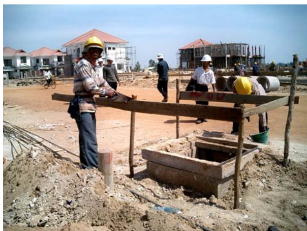
Figure 4. Improvement examples after participatory training; elevated workstation for farmers to avoid strenuous forward bending posture (left) and a guard to prevent falling down accidents in a construction site (right).
